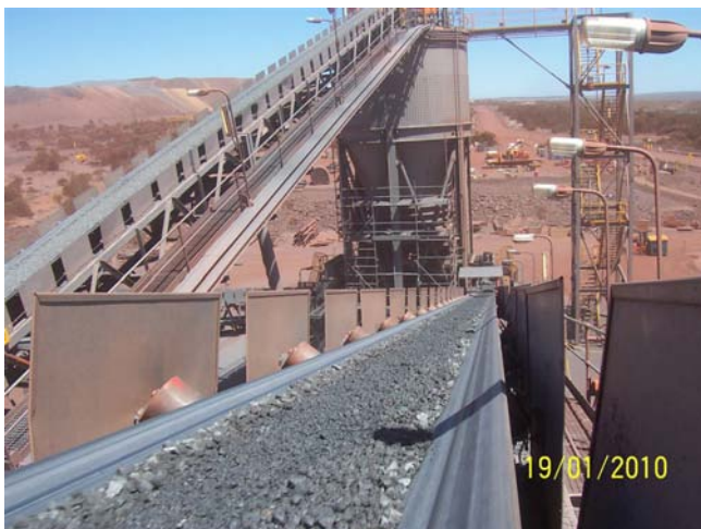
Photo 4 (Belt tracking to the LHS.)
