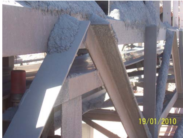
Photo 2 (Signs of insufficient belt tension in system.)
