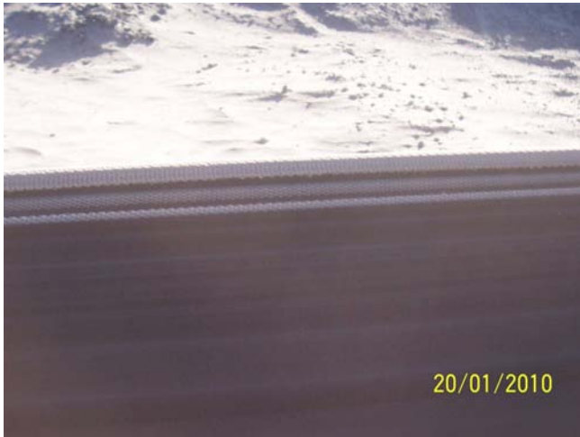
Photo 1 (Excessive edge wear to LHS to carcass.)
