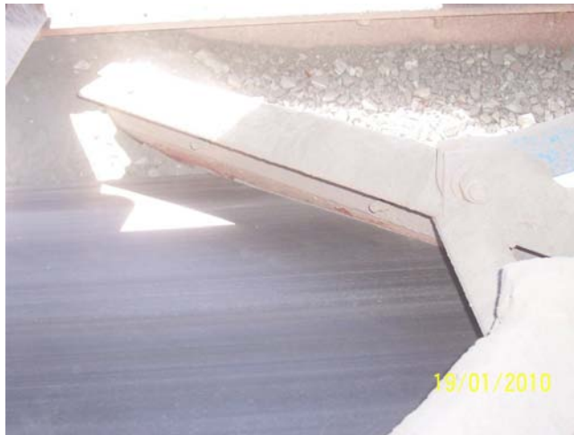
Photo 5 (Excess build-up on LHS/RHS of plough.)
