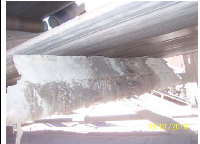
Photo 3 (Excess material build-up on cleaner at frame # 83.)
