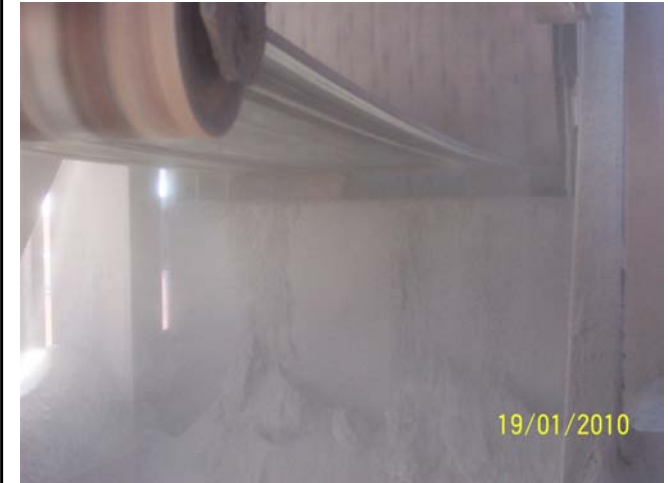
Photo 3 ( Excess material build-up under head pulley removed.)
