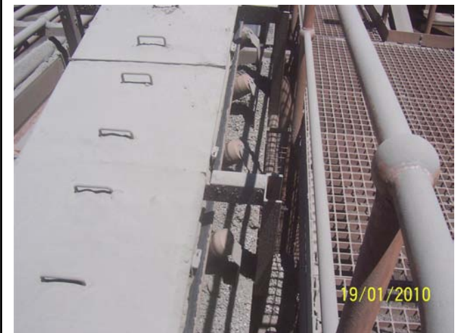
Photo 6 (Excess build-up around trough idlers LHS/RHS @ tripper chute.)
