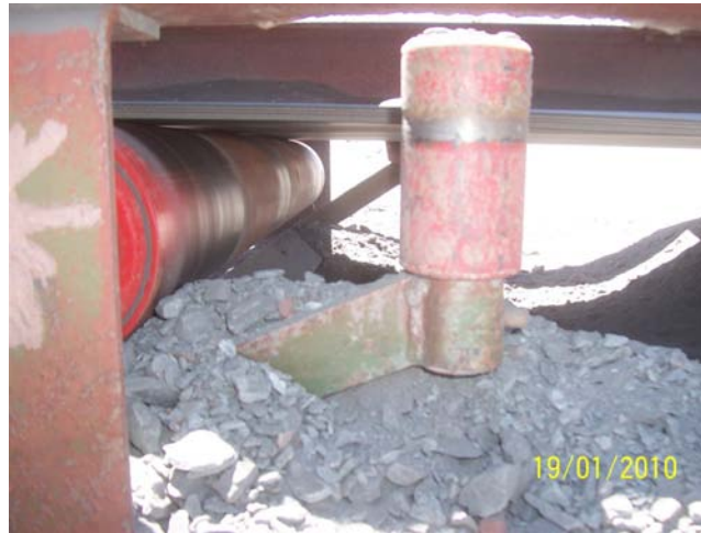
Photo 2 (Tracking frame buried at # 40.)
